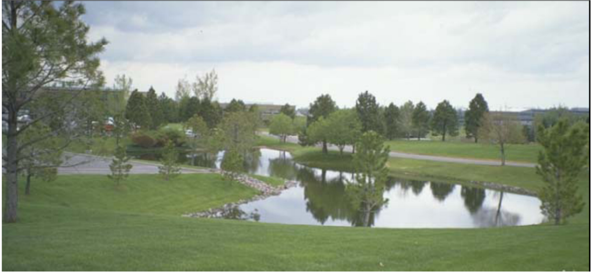
Fig. 60a – Bacia de retenção (EUA). Urban Drainage and Flood Control District, 2001.
